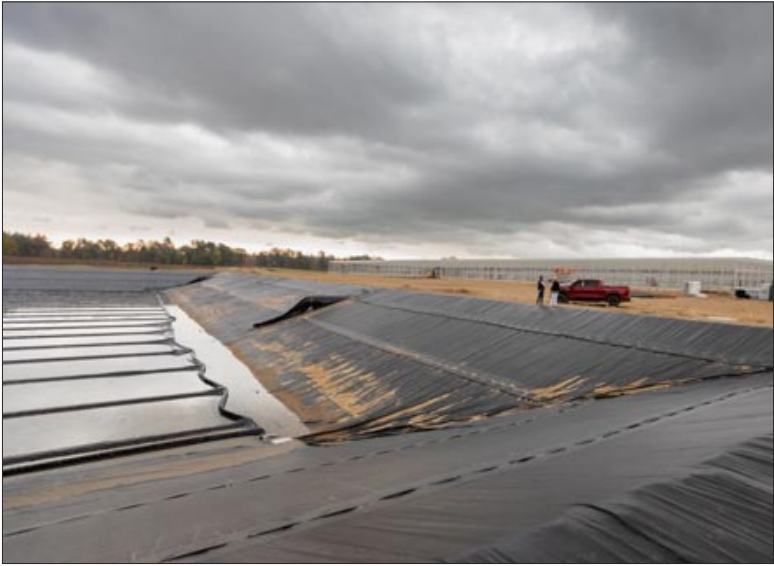
With emphasis on environmental stewardship, EZ Grow Farms has built a collection pond with capacity to store 50 million litres of rain-water that’s funnelled from the facility rooftops. As needed, the water can be filtered and recirculated through the growing facility.
